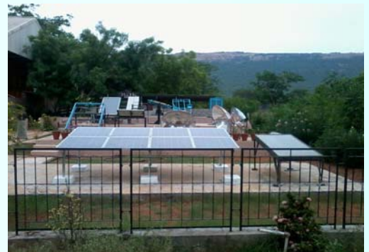
Test beds at Regional Solar Energy Testing Centre
