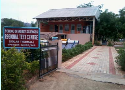
Regional Test Centre (Solar Thermal), MKU
